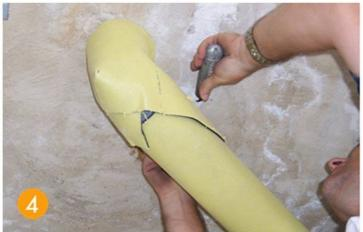
Measure and cutRemove nonstick paperStick to the tubeDuplicate in the curve
